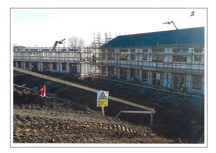
The steel frame has been constructed for blocks 1, 2, 3 and 4 and the floor slabs has been poured on the remaining two blocks 5 and 6.
